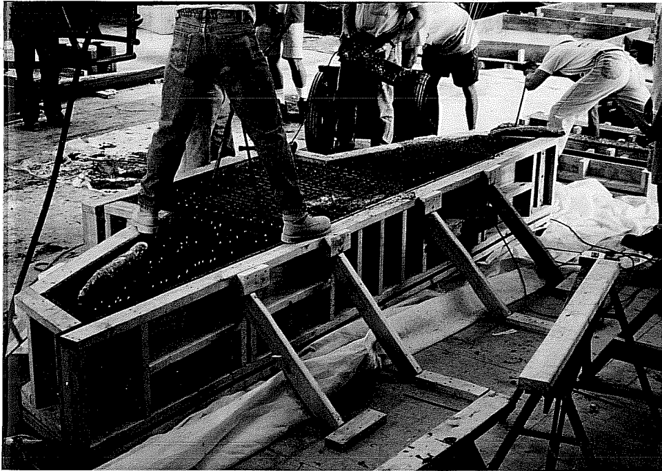
Figure 2.23 Formwork
